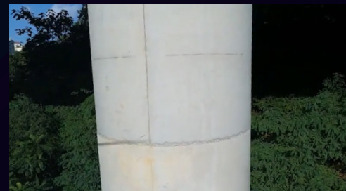
Inspection of bridge piers
