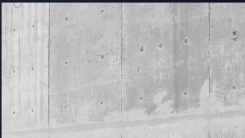
Inspection of Building Wall
